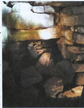
Looking into the creep passage
