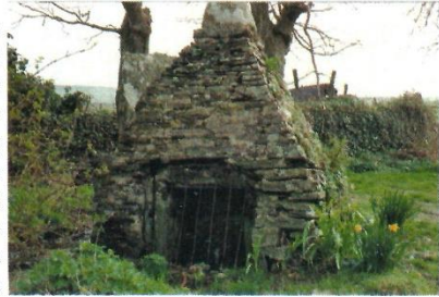
St.Perran's well at Trethevey
